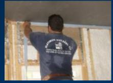
Foam gasket at ceiling/wall joints ensures airtightness
